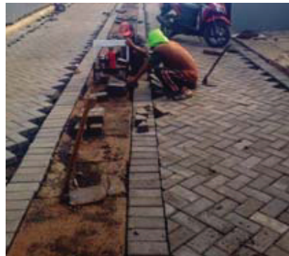
Sumber: www.cv-aditirtaaspalhotmix.blogspot.com Gambar 3.24 Tukang sedang memasang paving
