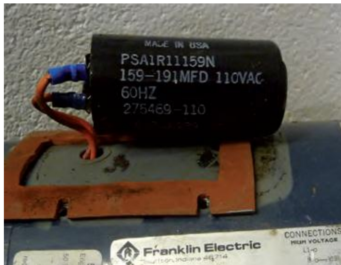
Gambar 5.3 Tipikal Starting Capacitor (159-191 mfd)
