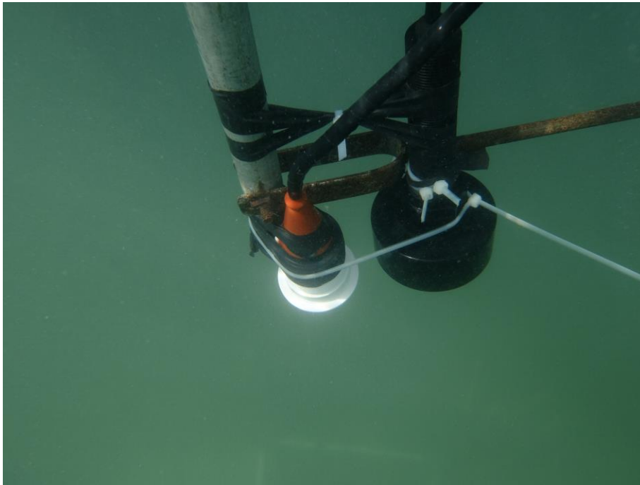
Underwater Transducer installation
